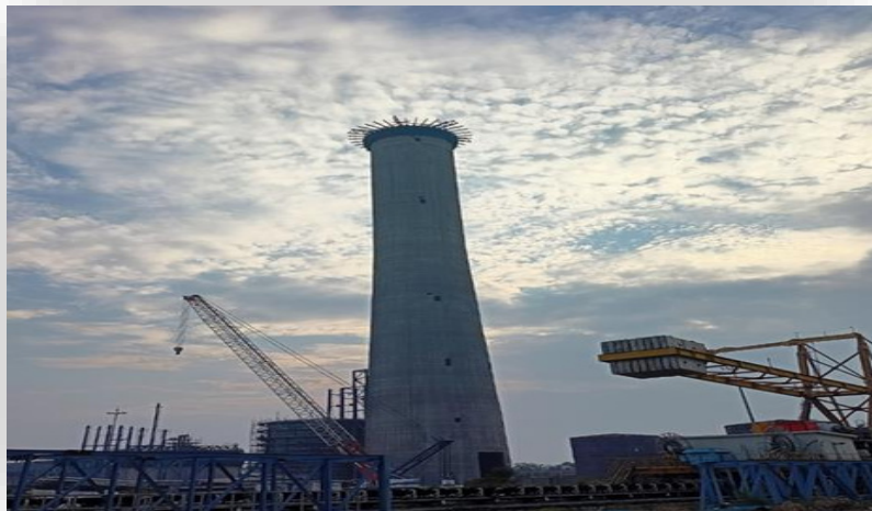
Wet Stack Shell Completed
