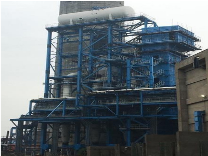
Recirculation Pump House
