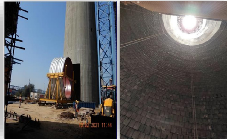
Borosilicate lining in progress
