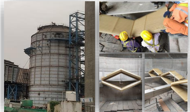
ME erection in progress
