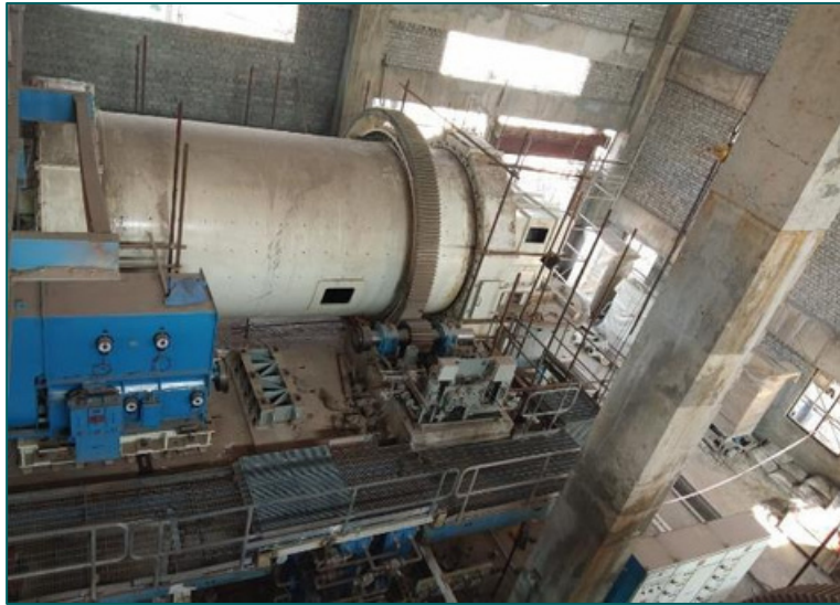
Ball Mill Building
