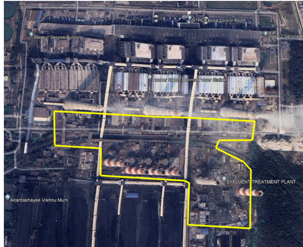
NTPC KANIHA (TALCHER, ANGUL DISTRICT, ODISHA) 6x500 MW FGD UNDER IMPLEMENTATION
