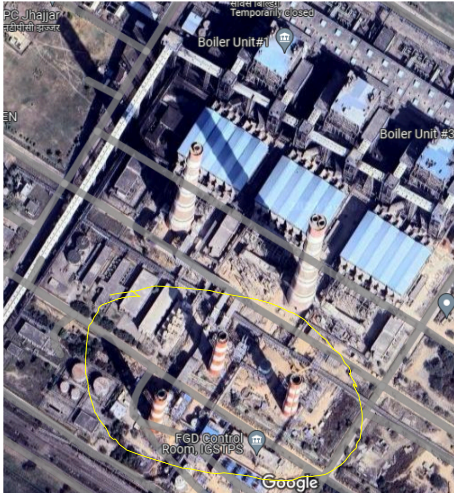
NTPC JHAJJAR STPP FGD SYSTEM
