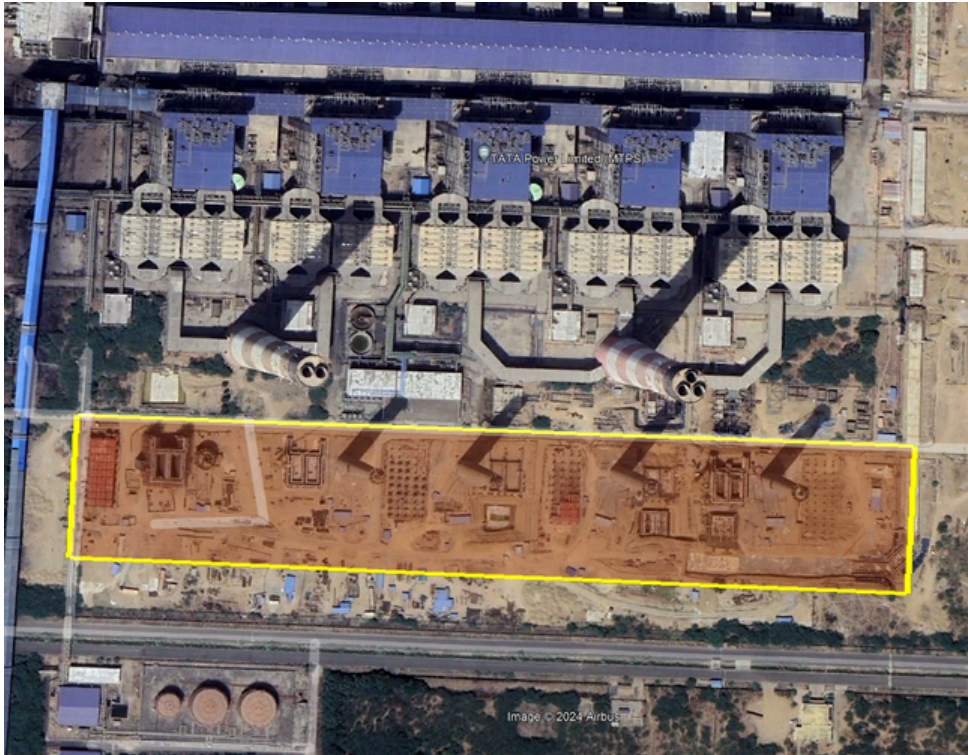
TATA POWER MUNDRA 5 UNIT STPP FGD UNDER IMPLEMENTATION
