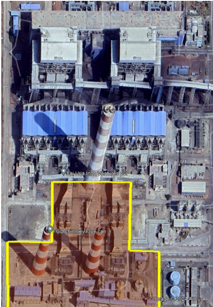
NTPC KHARGONE 2X660 MW STPP FGD
