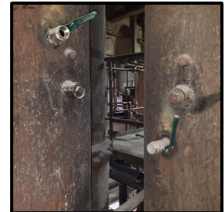
2 nos of provision made in coal pipe for flowmeter sensor fitting
