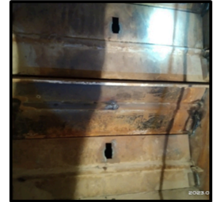
2 nos of provision made in coal pipe for flowmeter sensor fitting
